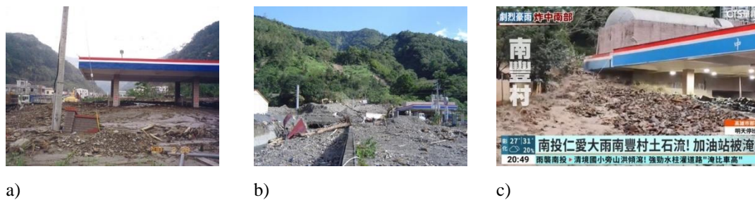
Fig. 2. St. Benedict (SB) gas station (No. “Touxian DF013” potential debris flow stream) in Nanfeng Village has been buried seven times by debris flows, making it the most buried building in Taiwan history [ARDWCT, 2023]: a – the first debris flow hazard at the SB gas station in the rainstorm in Feb. 2000 after the 921 earthquakes in 1999 (provided by J.D. Shieh on Feb. 28, 2000 [ARDWCT, 2023]); b – the sixth debris flow hazard at the SB gas station during Typhoon Sinlaku in 2008 (provided by S.C. Huang on Sept. 23, 2008 [ARDWCT, 2023]); c – Fifteen years later, from Aug. 3rd to 4th, 2023, Typhoon Khanun’s outer circulation caused the SB gas station to be buried for the seventh time by debris flow (from CTS TV image)
