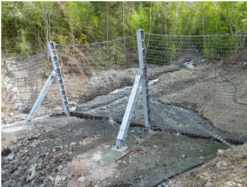
Fig. 7. Debris Catcher system from Trumer Schutzbauten (TS-DC-LAMBDA). Source: Trumer Schutzbauten
