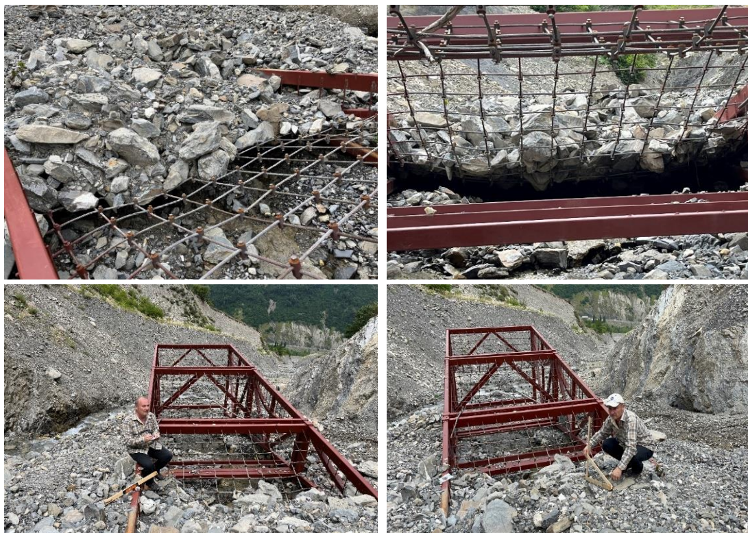
Fig. 9. General view of the debris flow regulation elastic barrage
