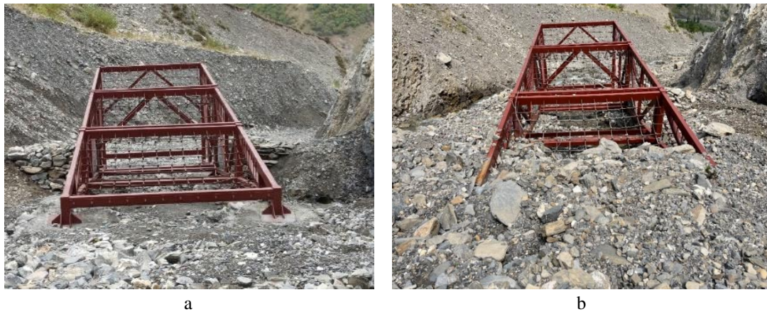
Fig. 8. General view of the debris flow regulation elastic barrage regulating solid fractions: structure before (a) and after (b) the debris flow passage
