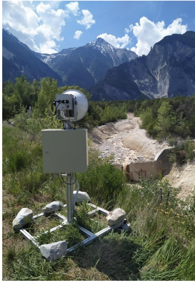
Fig. 1. PD radar installed at Illgraben. Check dam (CD) 27 can be seen in the background, where the stage sensor and range gate 2 are located
